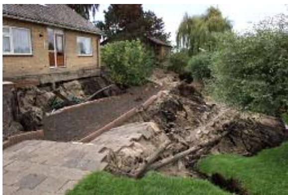
Fig. 6. Circular slip surface failure of the south-quay
