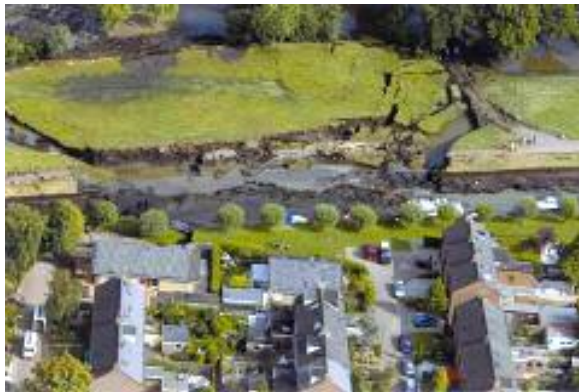
Fig. 5. Shifted part north-dike
